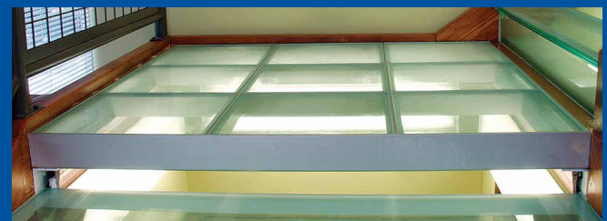
Total time for this stair landing: Approximately 2 hours
