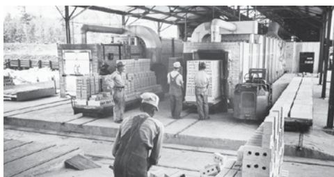
1960s kiln at Perla plant
