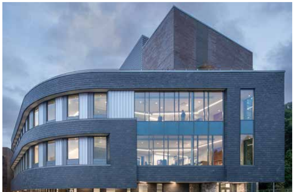
These cladding systems adapt natural slate to new architectural trends and styles that demand a more sustainable approach.
