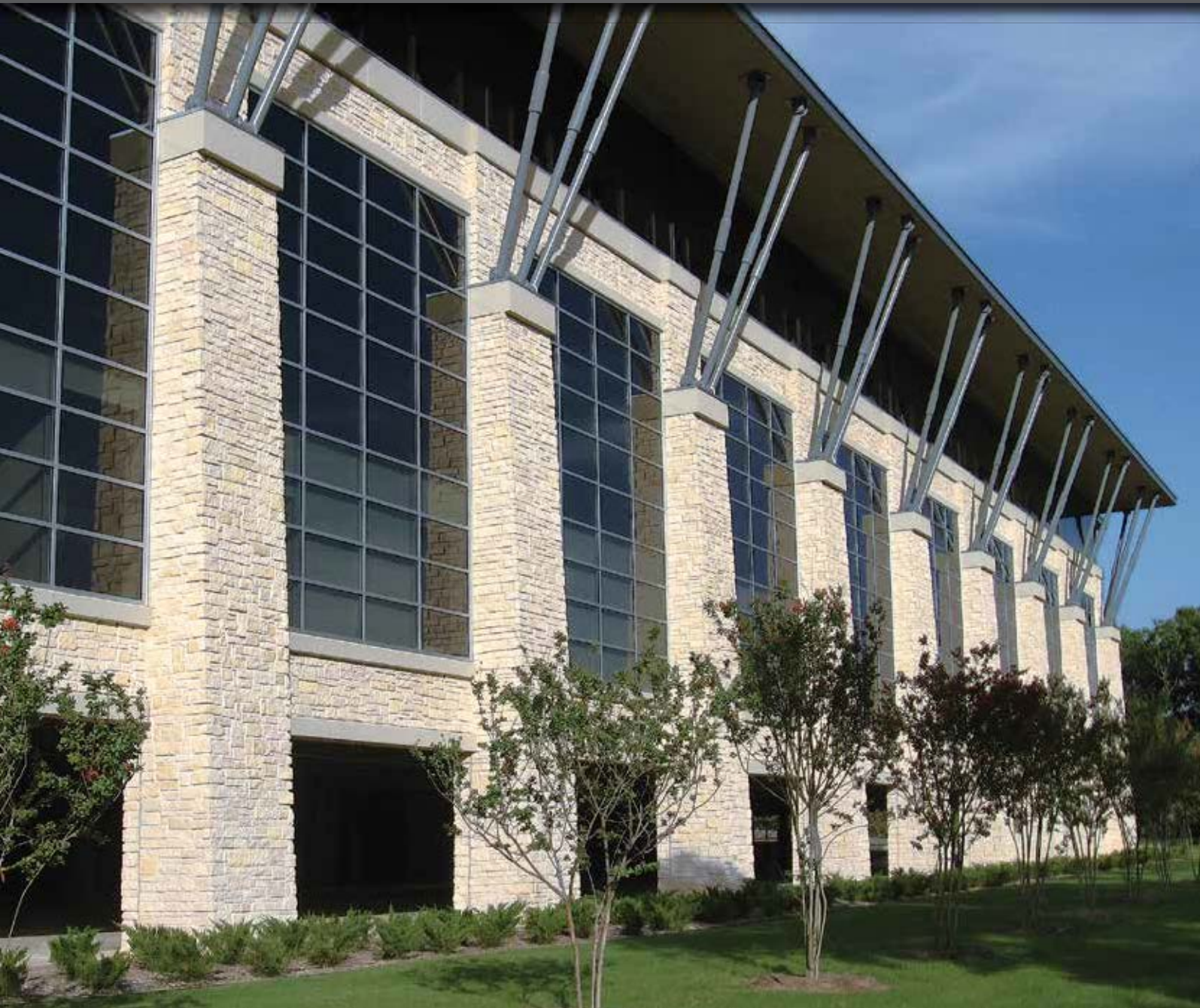
Texas Rubble - Texas Cream
