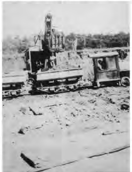
Loading a Perla rail car in about 1925 prior to the use of tractors and scappers.
