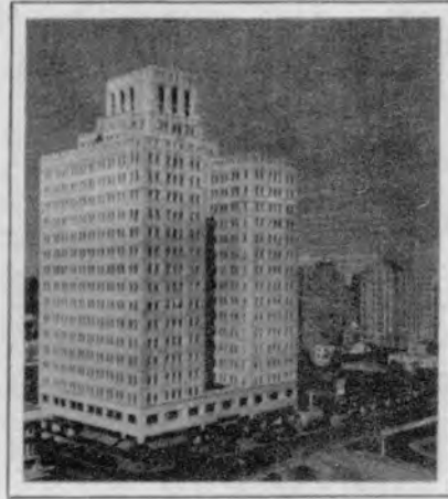
Faced with Varying Shades of Acme Ivory, Buff and Gray Face Bricks over Paris Blue
