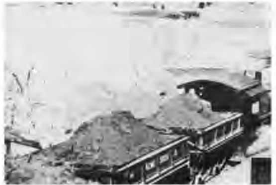
Acme steam trains hauled the mined clay to storage bins at the Perla plant. Most Acme plants went to the use of locomotives in the late 1920s and 1930s, but this system was used at Perla as early as 1924.
