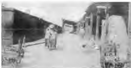
Worker is shown loading brick into boxcars by wheelbarrow at the Bennett plant in 1910. This method was used to load cars until the forklift came into use.
