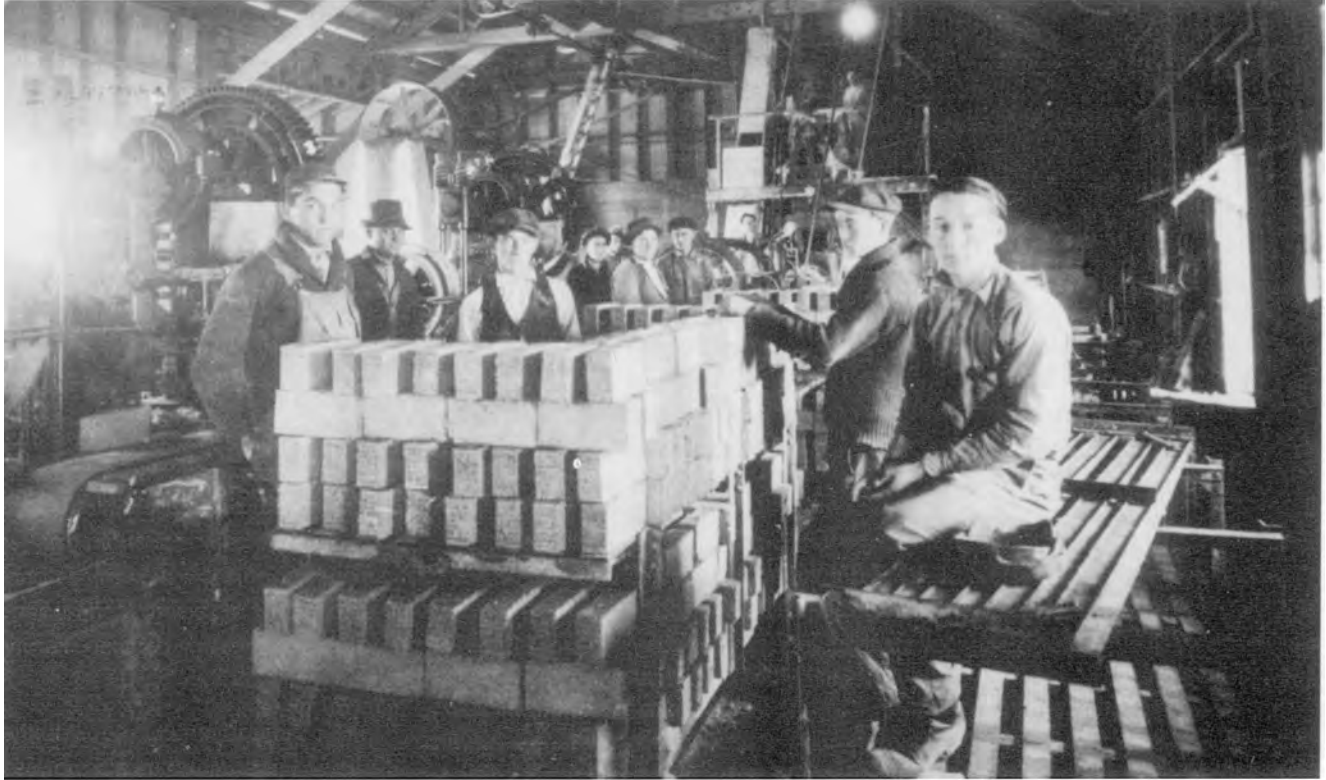
The inside of a machine room at Perla in 1931.
