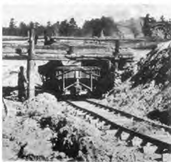
Loading clay into cars for delivery to a clay storage building. Tractors dumped the clay from above into hoppers that filled rail cars.
