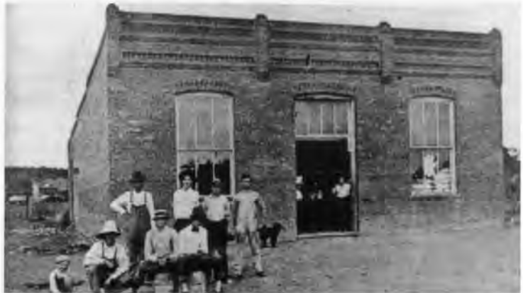
Right: Acme Pressed Brick's company store as it appeared in 1900.
