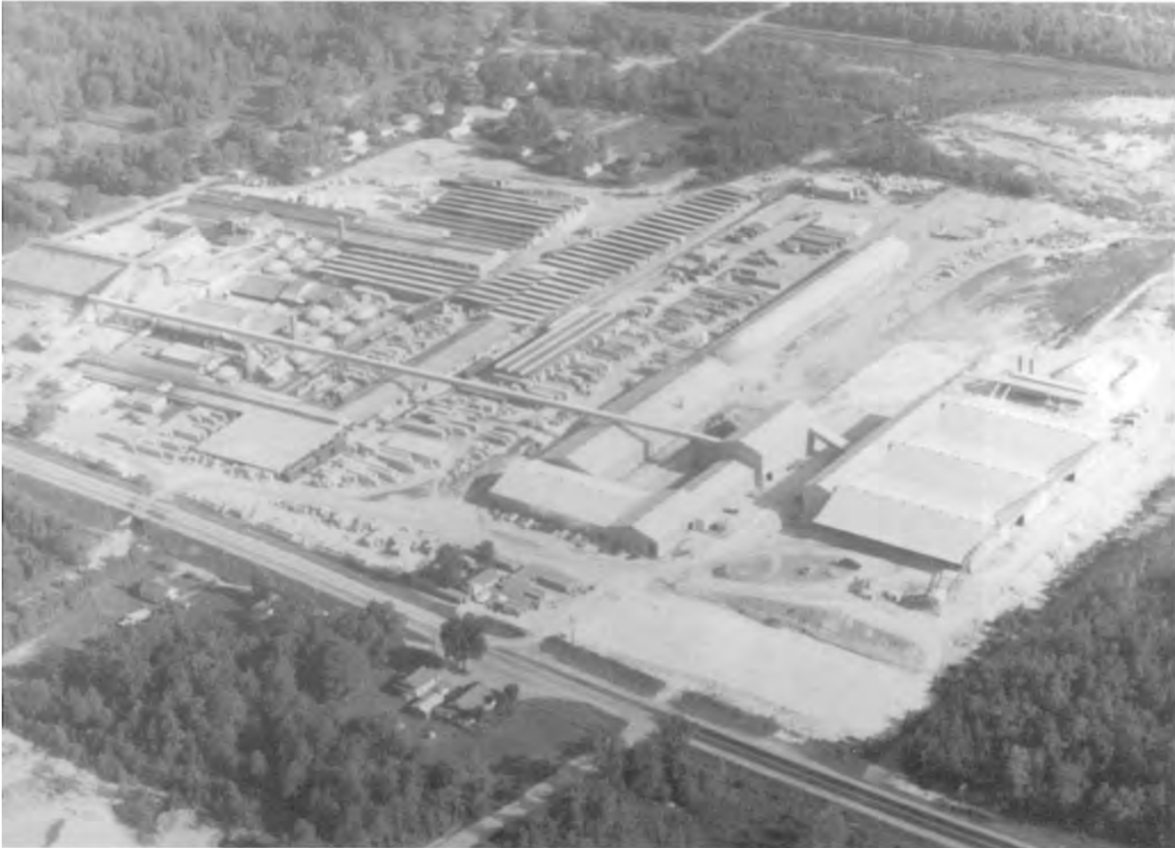
The Perla plant, an aerial view in 1968.
