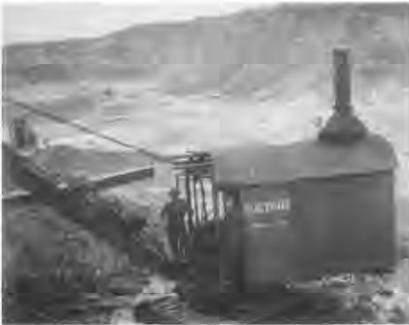
The Bucyrus steam shovel used at Denton prior to 1920. Such steam shovels were widely used to mine clay for brick plants until the late 1930s when they were replaced by diesel- and gasoline-driven machines.
