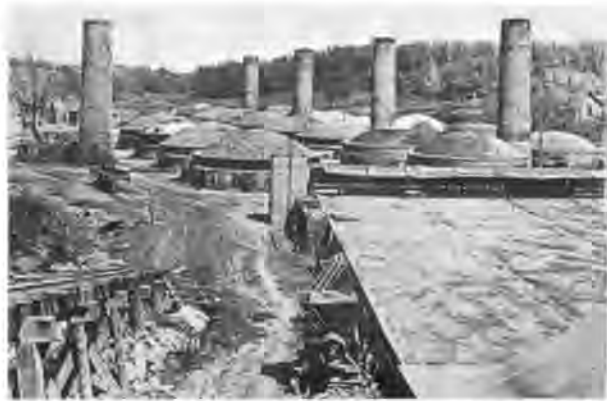
Acme's Fort Smith plant in 1921 as viewed from the railroad track that passed over a major public street that divided the pit area from the main plant. This situation exists today. Notice the company houses on the hill next to the plant.
