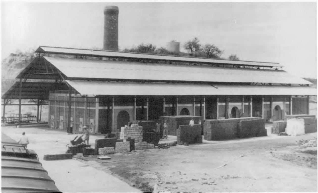
Bennett plant addition in 1956. These downdraft kilns increased the capacity by twenty percent.
