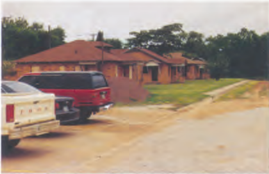
Experimental houses built with test brick just outside the Denton plant Research Laboratory in 1990.
