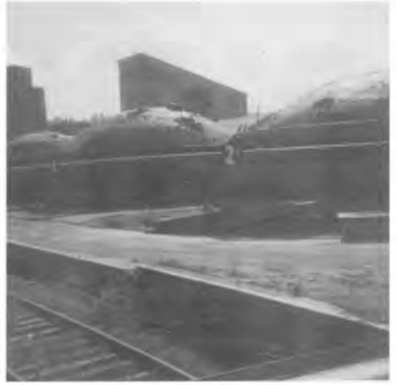
Left: An Acme Bennett plant kiln under repair for use in 1971. Note that it was metal banded then.
