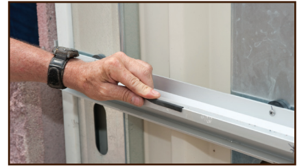
Flexible centering cushions are set on the lip of each channel...
