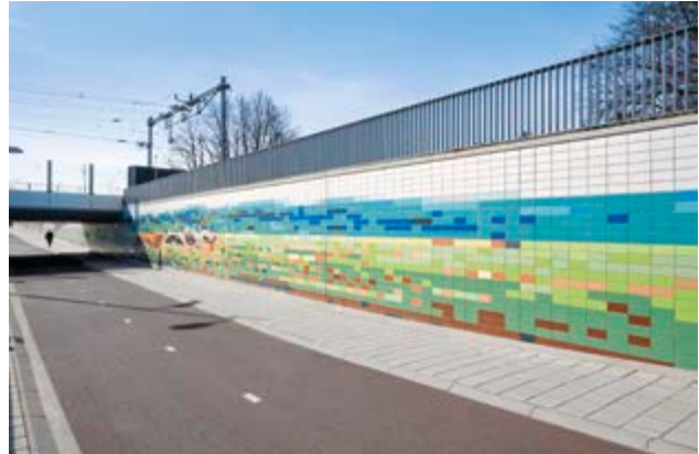
Effective where high levels of pollutants arise Fedor van Kregtentunnel, Netherlands / Architect: Royal Haskoning DHV, Mr Mari Baauw / Photo: Marcel van der Burg
