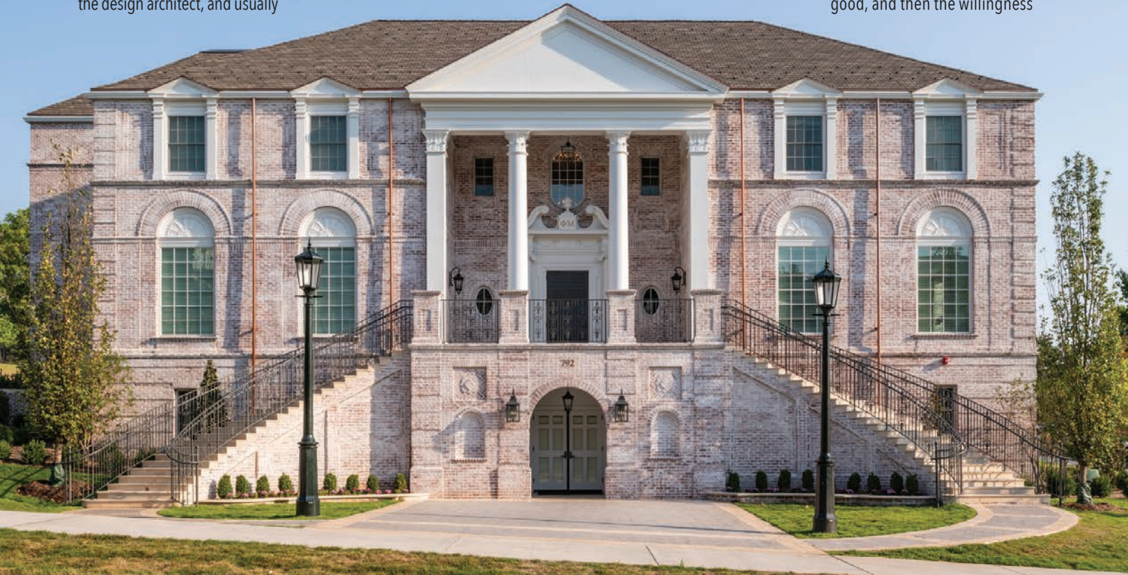
From architects' intricately detailed drawings, Acme Brick created special shapes and installation drawings for use in the field.
