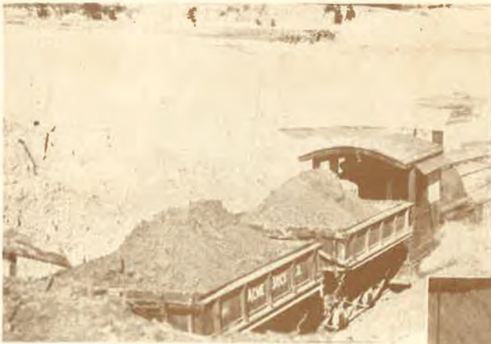
One of Many Acme Trains that Shuttle Between Pits and Mill
