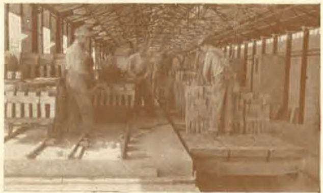
Setting the Tunnel Kiln Cars with Acme Brick just from the Dryer Cars
