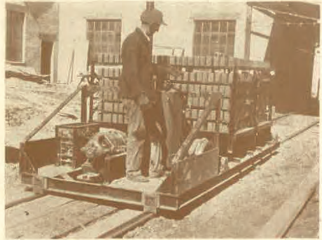
Transferring Brick from Tunnel Dryer Preparatory to Loading on Tunnel Kiln Cars
