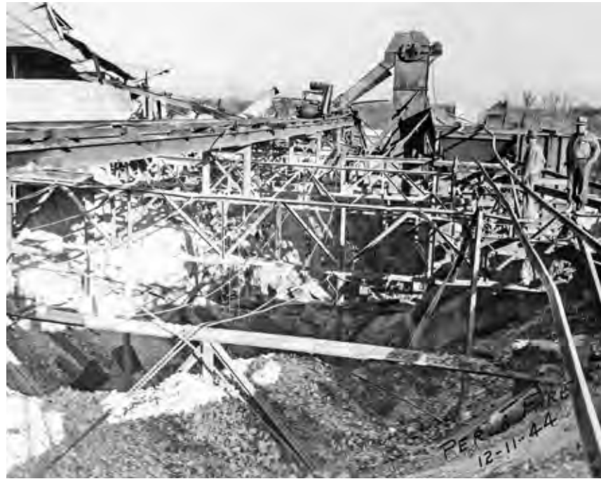
Supervisors stand on twisted girders and survey the damage after the fire at Perla on December 11, 1944.
