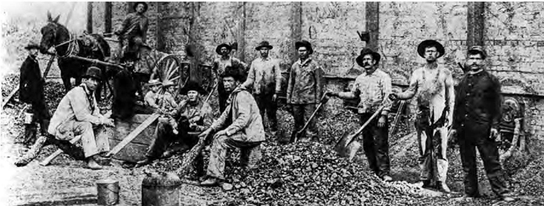
The updraft kilns had a voracious appetite for fuel, and shoveling coal to feed the kilns required sizable crews of men and mules to accomplish the task.
