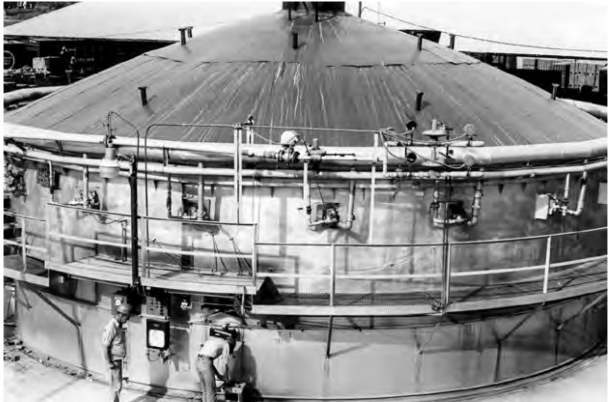
Workers perform kiln maintenance, circa the late 1950s.
