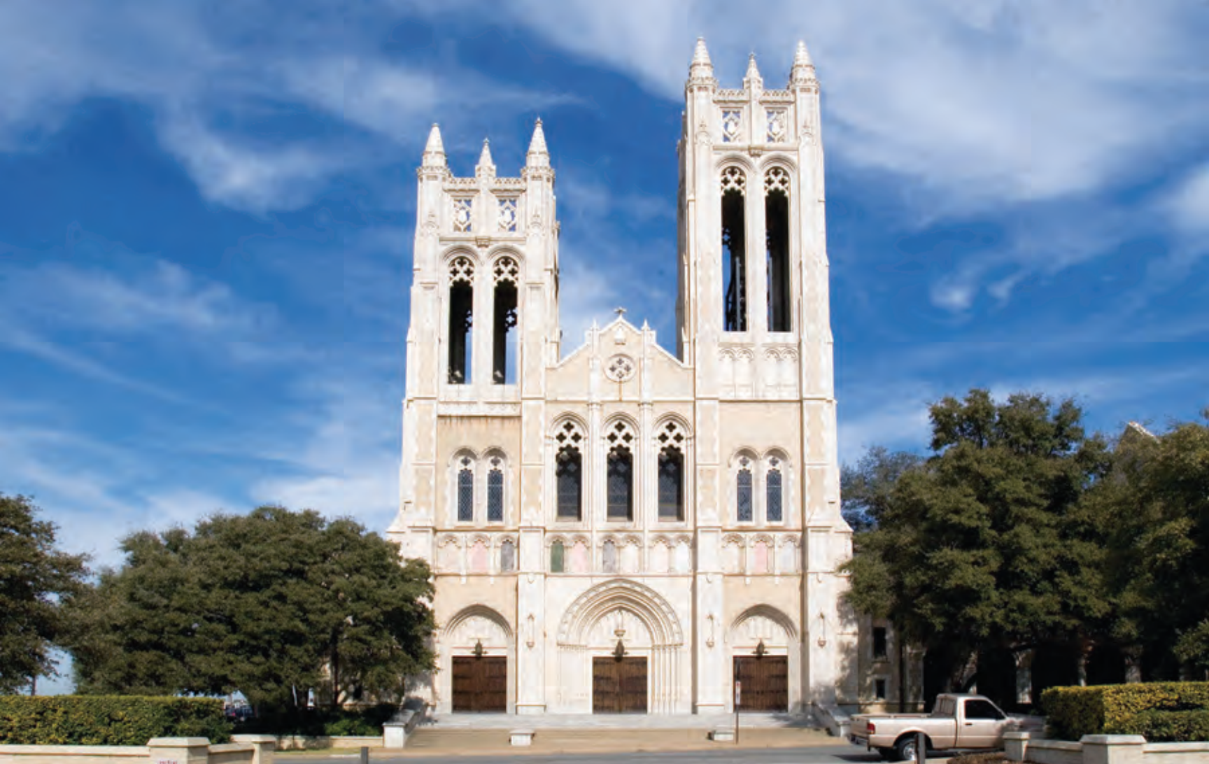
The Perla Brick used in the construction of the United Methodist Church in Fort Worth shone as bright in 2005 as when it was installed in the 1930s.
