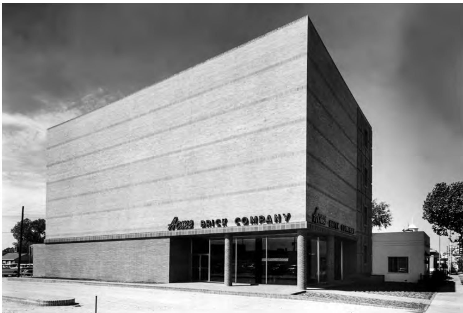
Acme Brick's newly completed Fort Worth Headquarters on Seventh Street in 1952.
