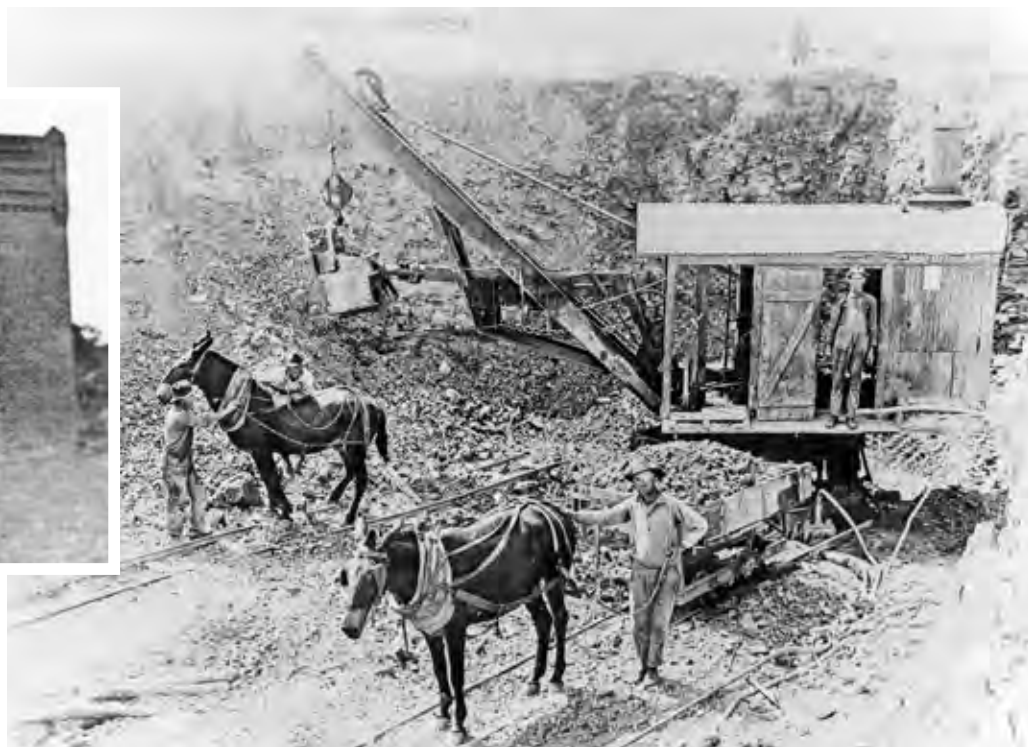
A steam-powered shovel fills rail cars pulled by mules with shale at the Denton mining pit, circa 1900.
