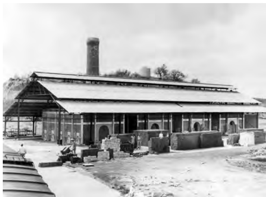
The 1956 Bennett Plant addition; the downdraft kilns pictured improved production by 20 percent.
