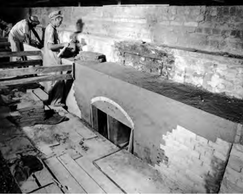
Masons repairing a kiln in the 1940s.
