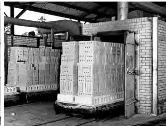
Above: White Brick emerging from a kiln at the Perla Plant in 1949.
