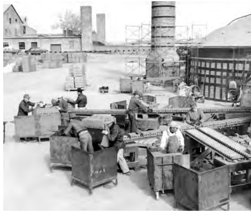
Above: A worker pours a mold from a one-hundred-pound sack of refractory concrete sometime in the early 1950s.
