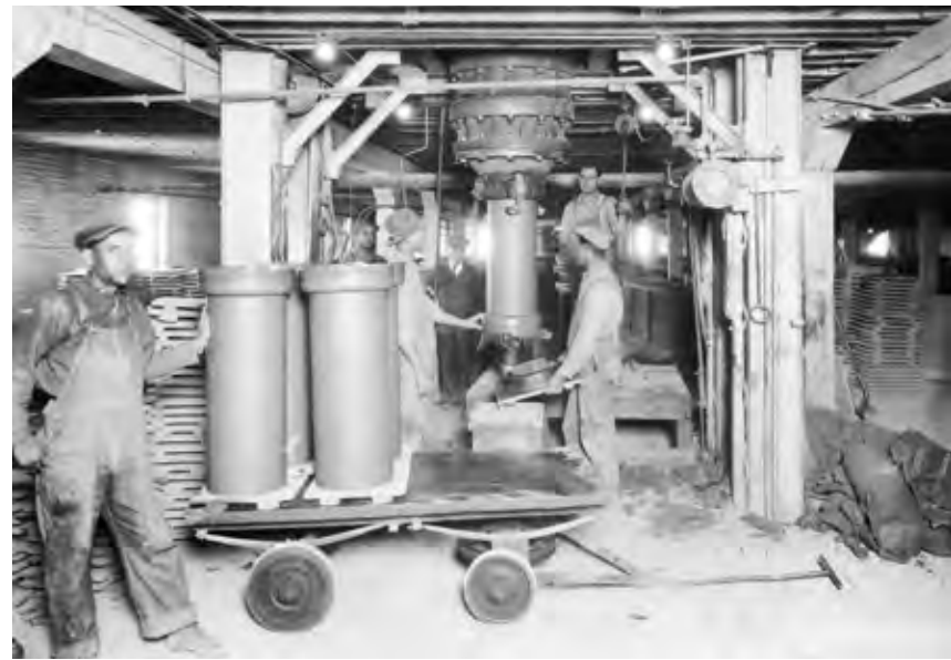
In about 1915, these workers extruded unfired sewer pipe at what is now Acme Brick's Plant near Denver, Colorado.
