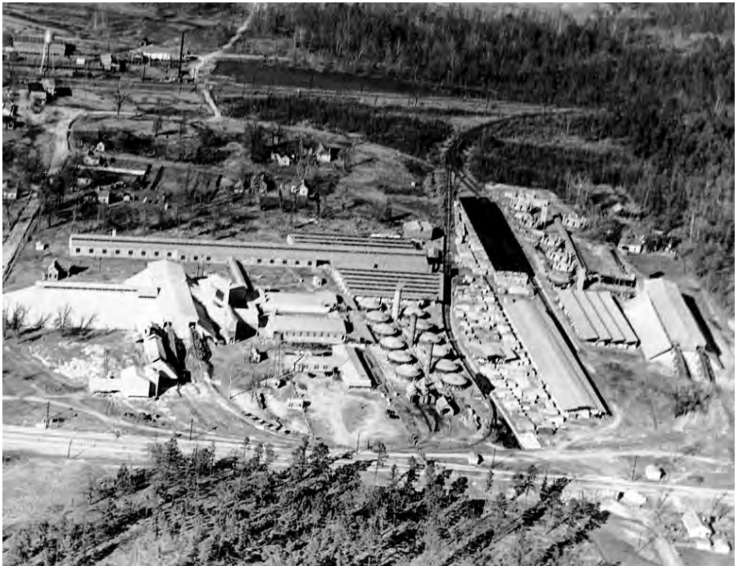
This postwar aerial view of the Perla Brick Plant with tunnel kiln and beehive kilns indicates that brickmaking had changed little since early in the twentieth century.
