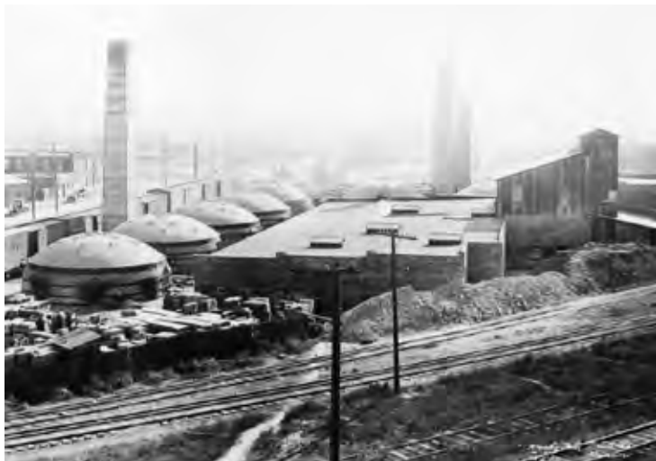
A typical plant layout in the 1920s showing round kilns to the left and the importance of a rail siding in the foreground.
