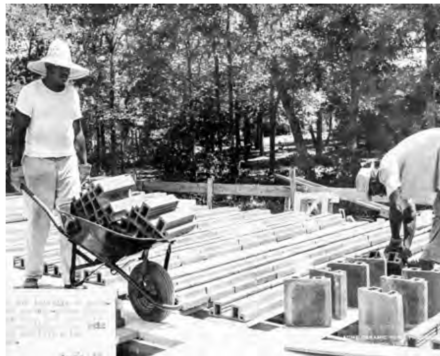
Following World War II, Acme Brick heavily promoted the building of ceramic homes, seen here at two homebuilding sites in Austin in 1949.
