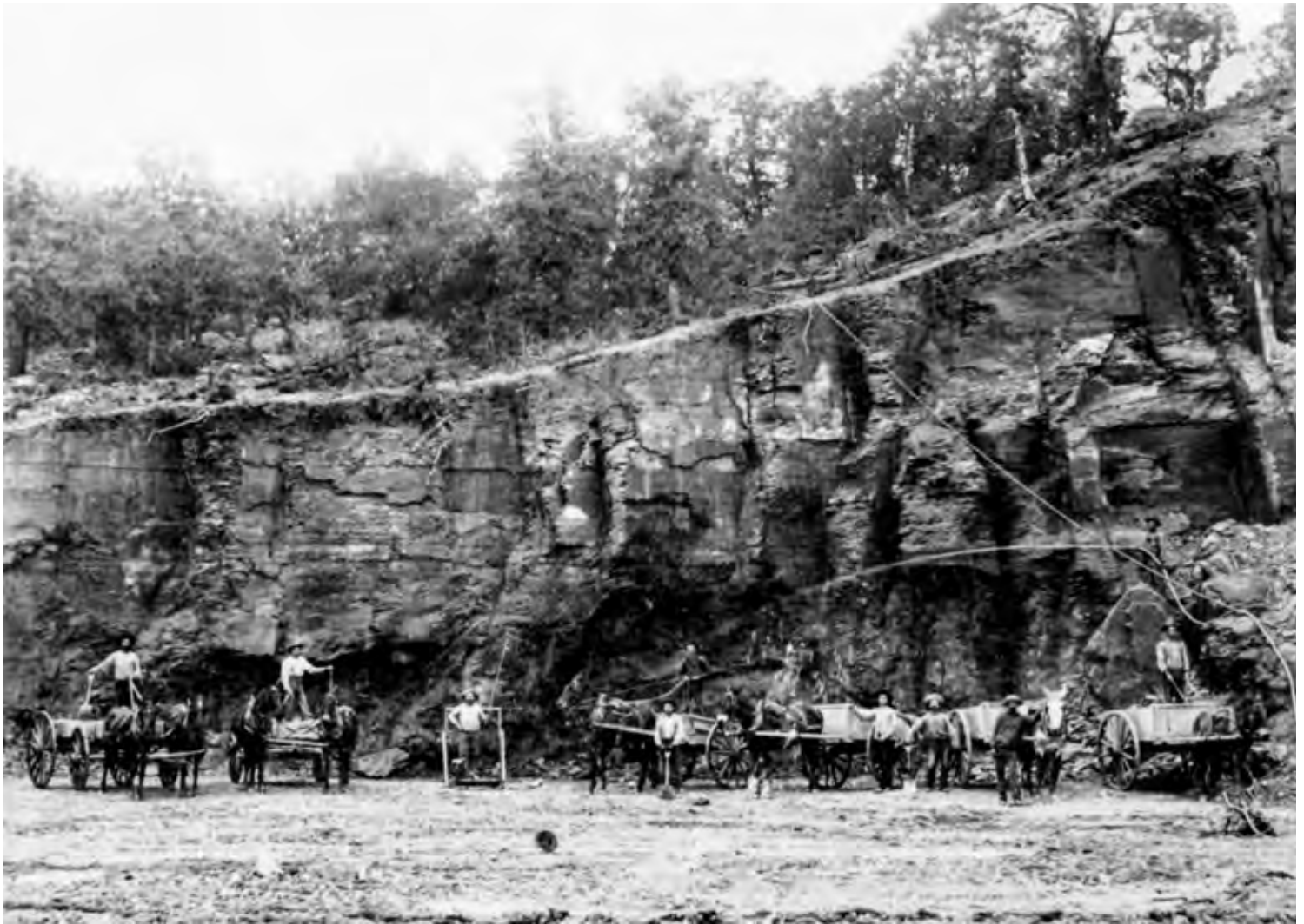
In the days before heavy equipment became commonplace, men with picks and shovels worked at the face of the shale deposit, loading shale into horse-drawn wagons, like here at Bennett in the early twentieth century.
