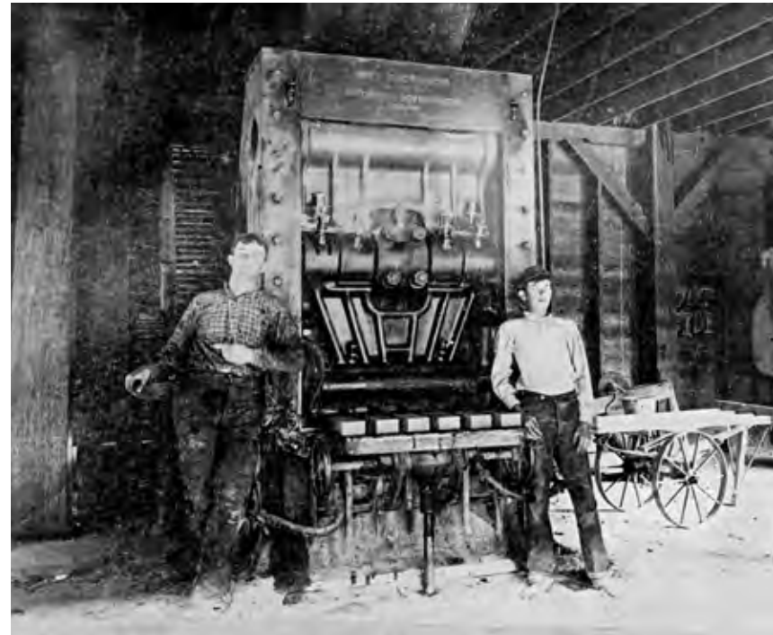
Above: This Boyd Six-Mold Press installed at the Bennett Plant in the 1890s helped to dramatically increase the efficiency of the production line.
