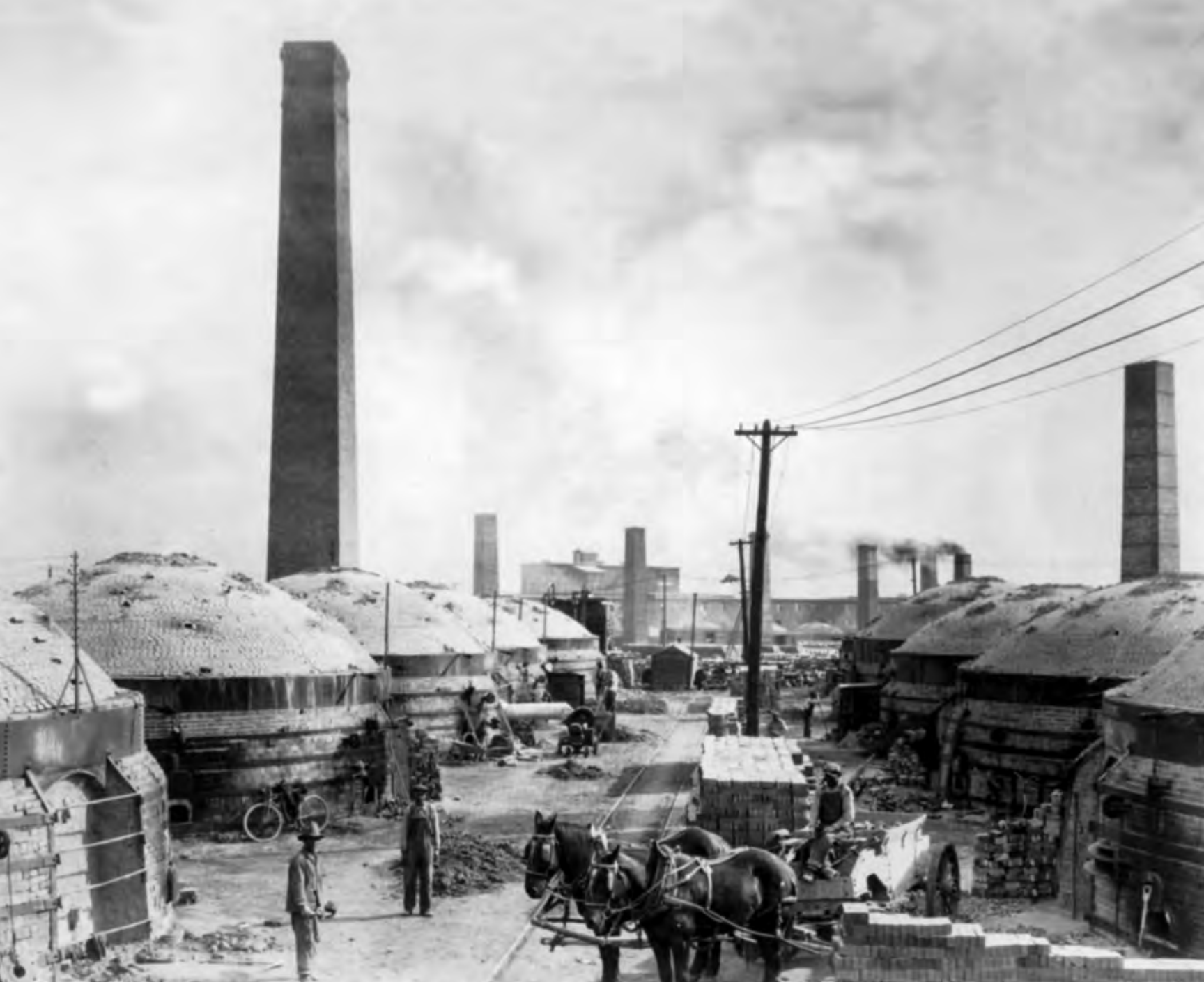
By the 1920s, electrification of the brickmaking process was well under way at the company's Denver Plant.
