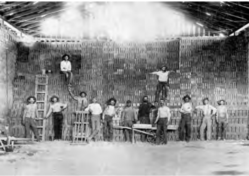
In the Bennett Plant's updraft kilns, brick were carefully hand-stacked for the most effective firing.
