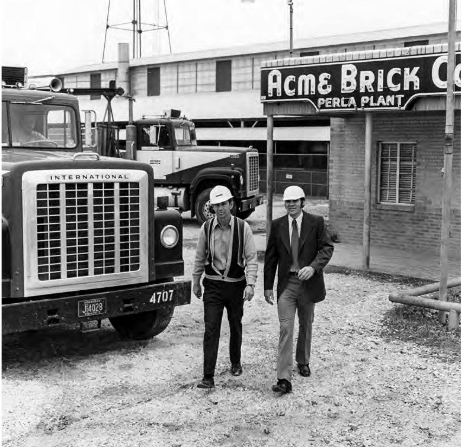
An Acme Brick salesman (right) visits the Perla Plant in 1973.
