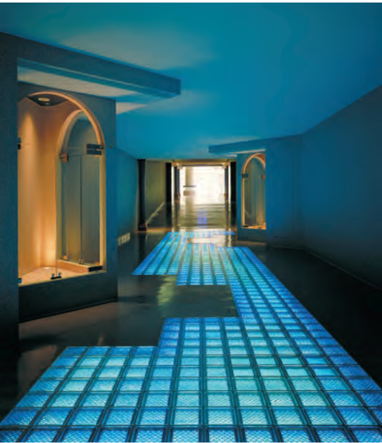
In this 1999 Innovative Building Products installation at LeBonheur Childrens' Hospital in Memphis, Tennessee, lighting beneath the IBP floor system gives the appearance of water rippling underneath the glass pavers.
