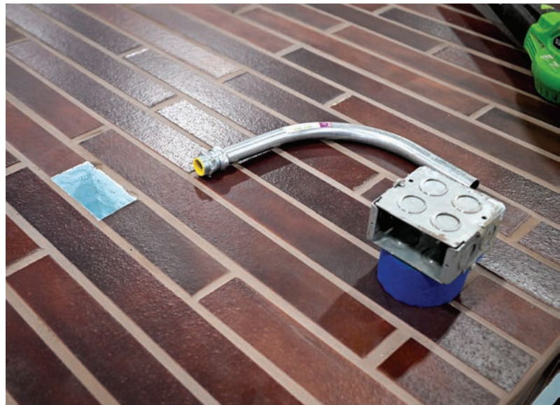
Thin brick slips are installed by BakerTriangle on prefab panels destined for Fred Hill Elementary School.
