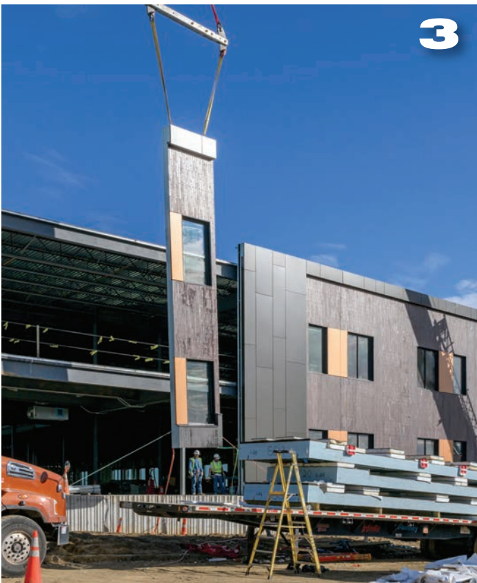
Installation of prefab panels at Fred Hill Elementary
