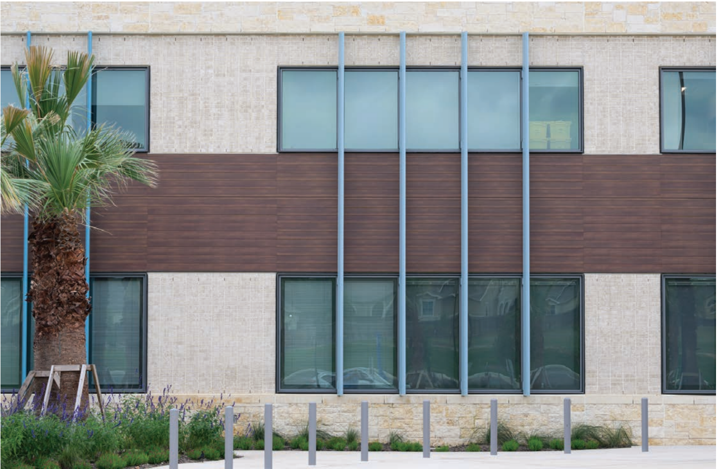
Brick to Limestone Transition. See Section Below.
