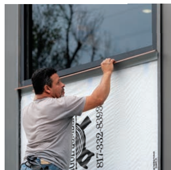
header install over vapor barrier
