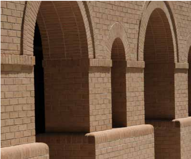
Bullnose Soldiers, large 2 piece stacked roman arch, small single piece roman arch.
