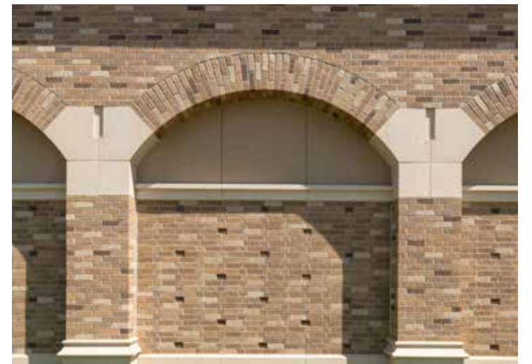
Segmental multi piece arch, and field wall with inset turned brick.
