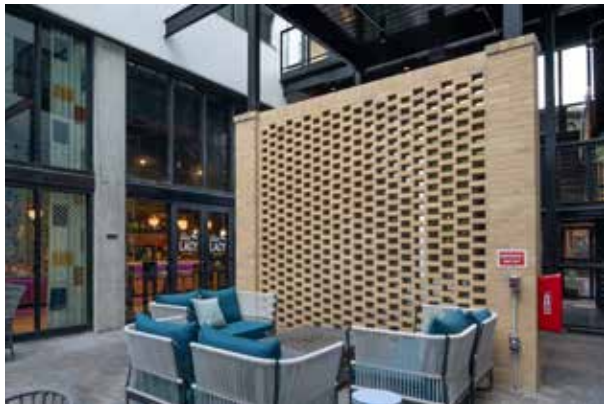
Screen wall created with solid modular brick offset.
