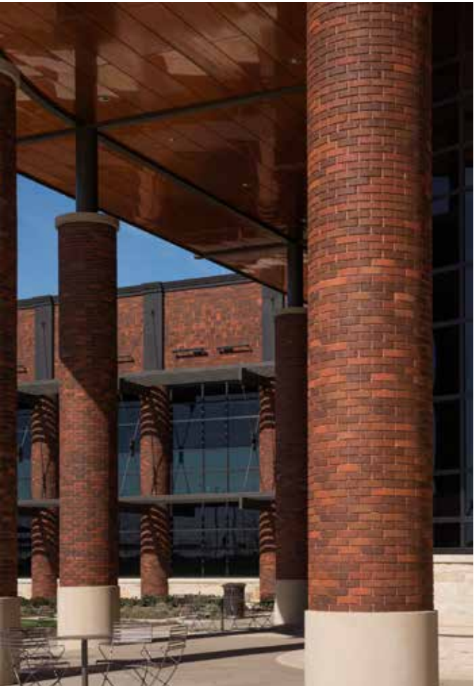
Radial brick columns.
