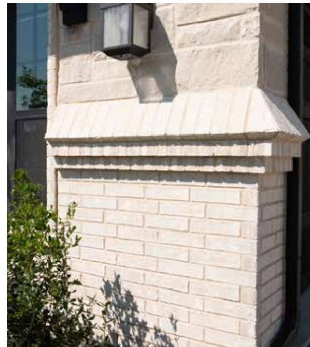
Custom detailing, with sloped soldier brick.
