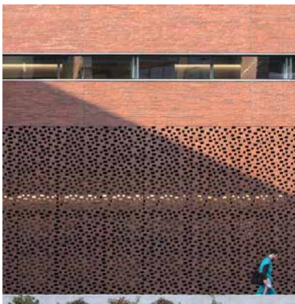
Screen wall created with norman and cut brick.
