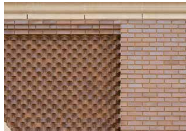
Inset of field brick turned 45 degrees.
