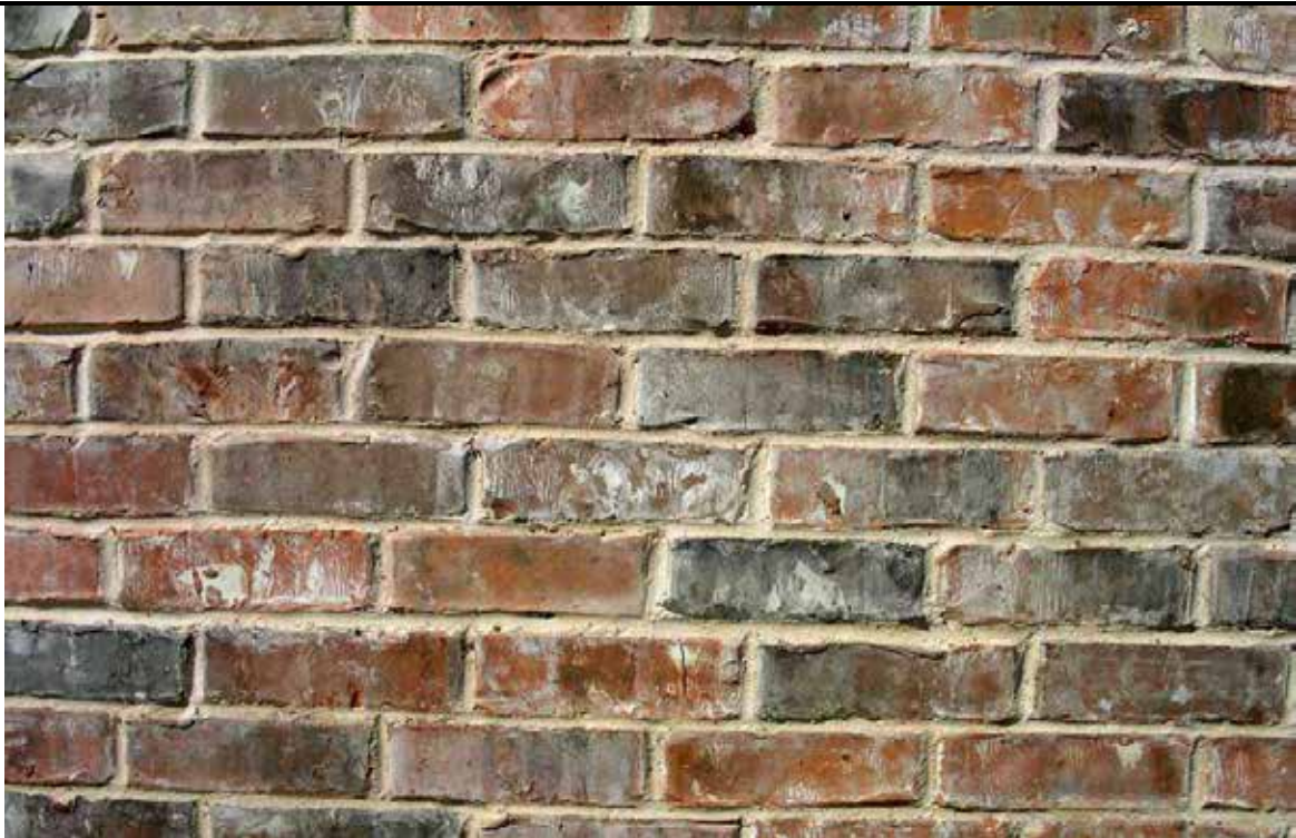
Figure 1. Brickwork with dryer cracks viewed five feet away. At twenty feet they are not visible.
