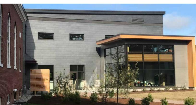
offer thermal insulation, prevent excessive air leakage and carry wind loading. The slate actually breathes just like a skin, as the inner layer reduces energy losses.
