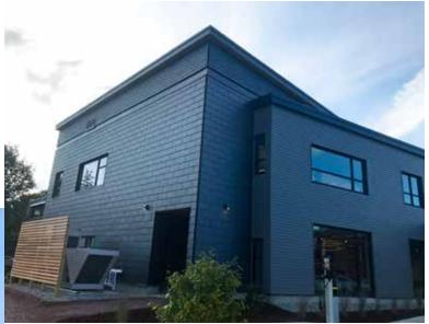
"One major challenge was because the walls of the library were tall, we were apprehensive about load bearing factors. And because the building was designed with a Net Zero energy, exterior envelope of 4" thick insulation, the weight of the façade was a concern," Nedzinski continued. "The installation process was researched, and ultimately by crossing layers of z-girts, the CupaClad<sup>®</sup> system was successfully adhered to the building's exterior."
