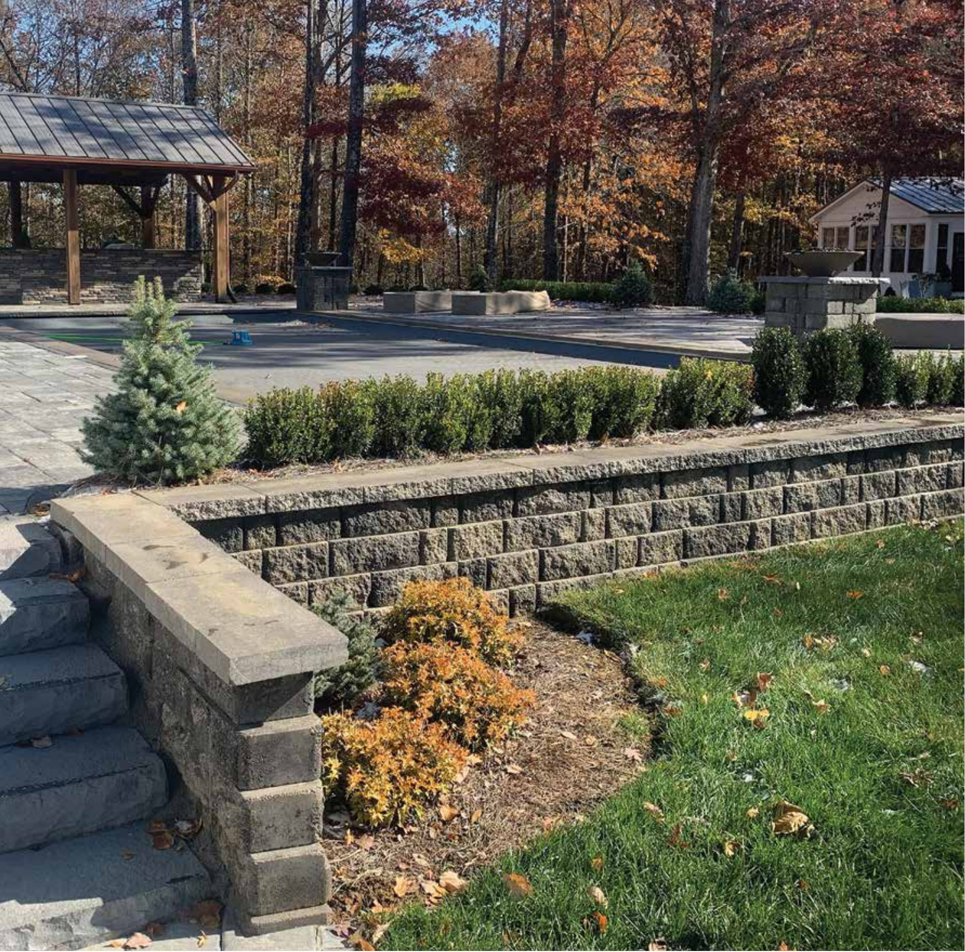
Harington - Medley offers a combination of scored and straight split units achieving the beauty of a three-piece system with the efficiencies of a single unit installation. The rear lip simplifies alignment and speed of construction.
