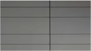
Stack horizontal installation
