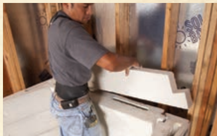
2. Starting the smoke chamber
