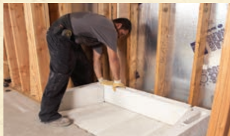
1. Installing base and first course
