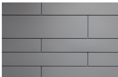
Horizontal counter-joint installation
