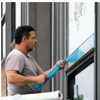
removal of protective film
