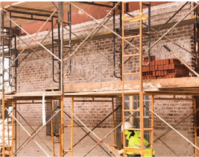
An initial sack finish was applied by masons as the wall went up, and then a second pass near completion brought the unique appearance to the character approved by architects on-site.
