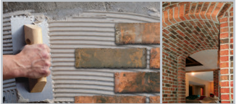
Interior or exterior mortar application on masonry or concrete.
