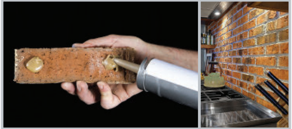
Adhesive interior installation on wood/steel stud framing.
