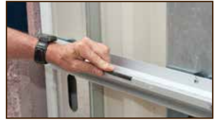
Flexible centering cushions are set on the lip of each channel...
