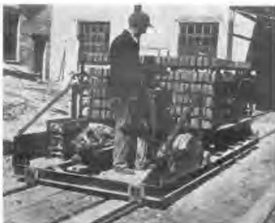
Dried brick being moved to be loaded onto kiln cars in 1930.
