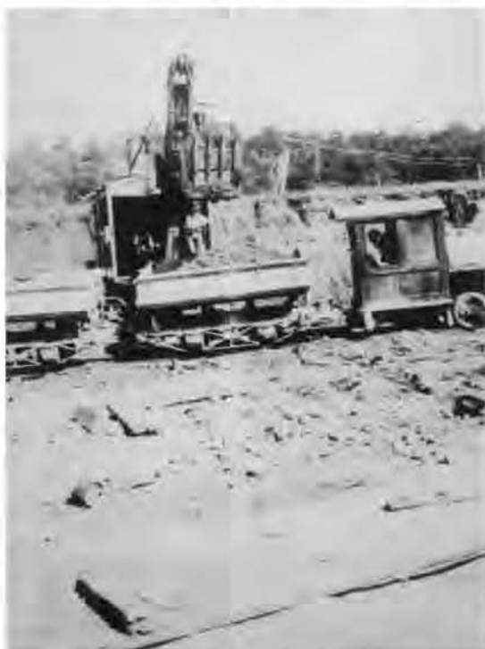
Loading a Perla rail car in about 1925 prior to the use of tractors and scrappers.
