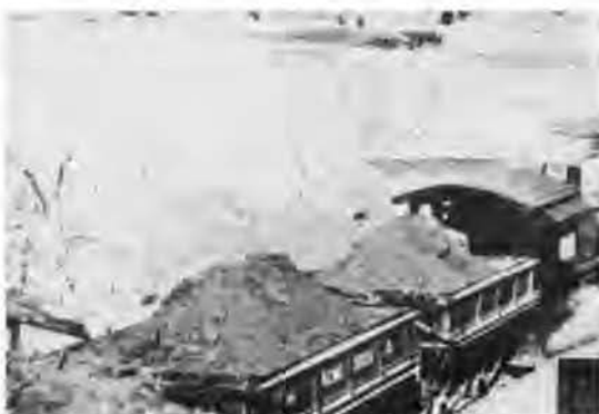
Acme steam trains hauled the mined clay to storage bins at the Perla plant. Most Acme plants went to the use of locomotives in the late 1920s and 1930s, but this system was used at Perla as early as 1924.
