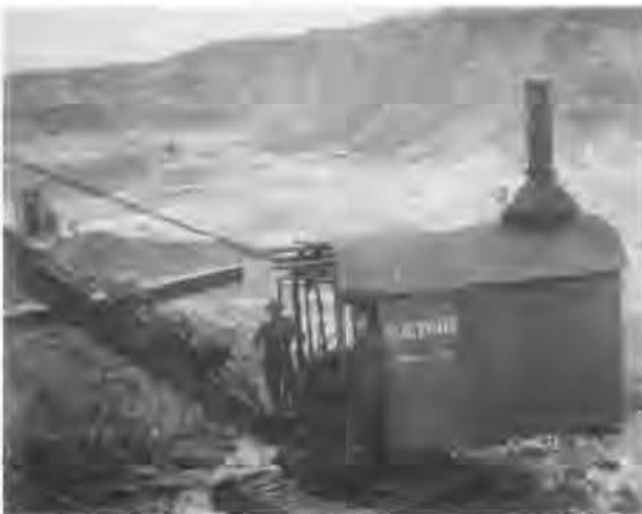
The Bucyrus steam shovel used at Denton prior to 1920. Such steam shovels were widely used to mine clay for brick plants until the late 1930s when they were replaced by diesel- and gasoline-driven machines.
