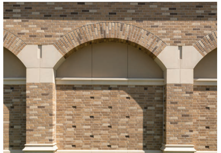
Segmental multi piece arch, and field wall with inset turned brick.
