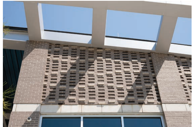
Slate Gray modular wall with inset dark gray brick, popped out light gray brick.
