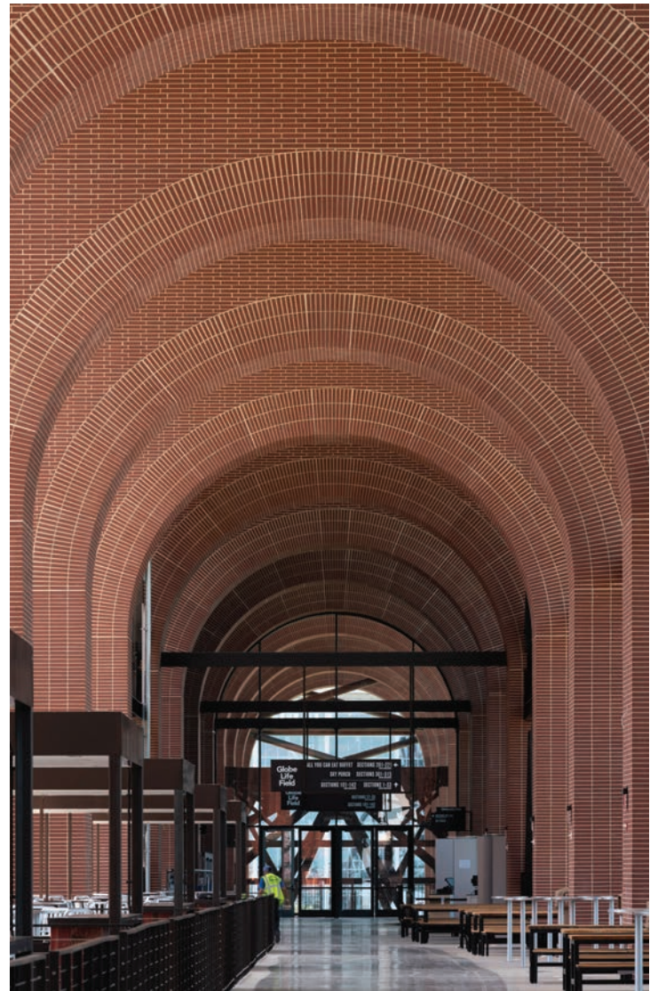
This arch has such a large span, that it is achieved with stacked norman size field brick. The mortar between each is tapered.
