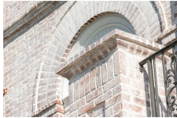
Roman stacked three piece arch in background, with a column in foreground with soldiers and ogee shapes.
