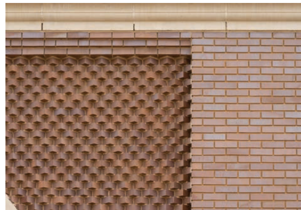
Inset of field brick turned 45 degrees.
