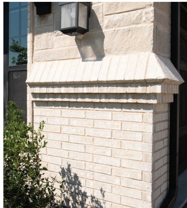
Custom detailing, with sloped soldier brick.
