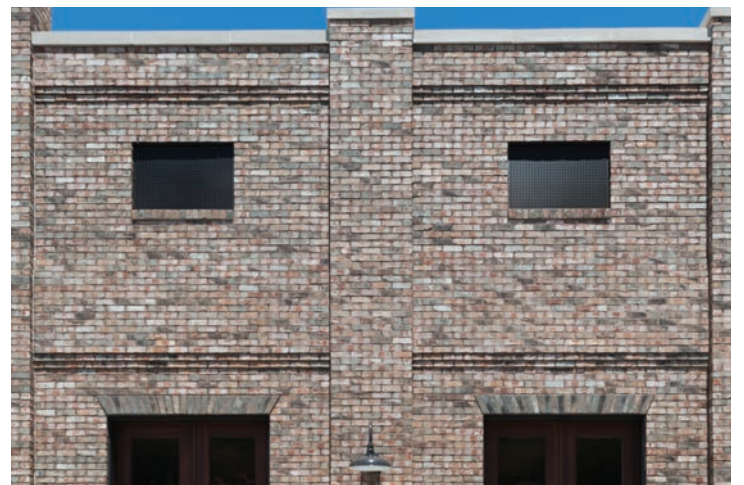
Window sills of face brick, single piece jack arch over doors.
