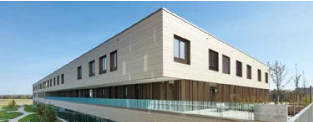
Medical day care unit ZfP Südwürttemberg, Biberach, Germany Architect: Die Ulmer Architekten BDA / Year: 2020 / Photo: Conné Van D'Grachten
