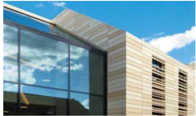
Raiffeisen Forum, Mödling, Austria / Architect: arge x42 / Year: 2014 Photo: Rich Hiebl
