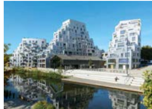
Ilot de l'Octroi, Rennes, France Architect: MVRDV, Rotterdam, the Netherlands
