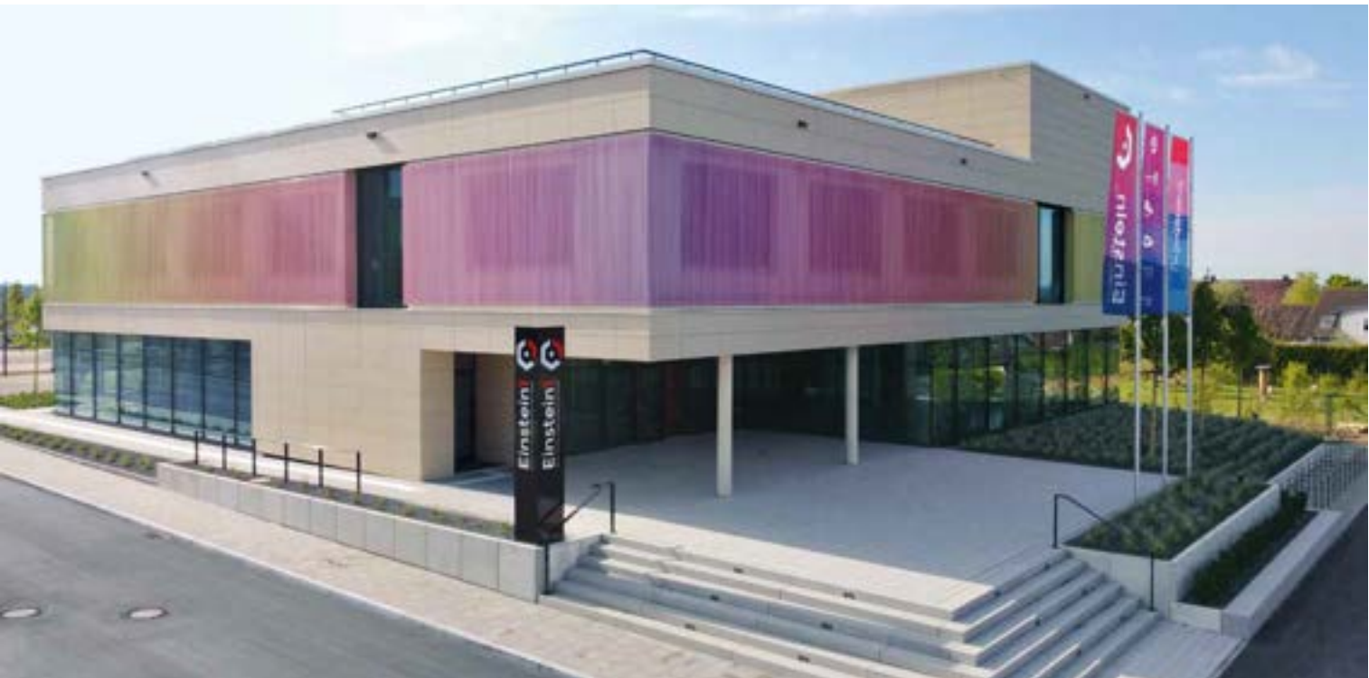
Start-up centre "Einstei 1" at the campus of HAW Hof, Germany / Architect: Architektur GmbH (Renee Lorenz) / Year: 2019 / Photo: Vanessa Wagner
