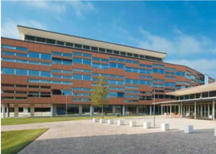
Green Life Headquarters Banca Crédit Agricole, Parma, Italy / Architect: Frigerio Design Group / Photo: Frigerio Design Group / LEED PLATINUM
