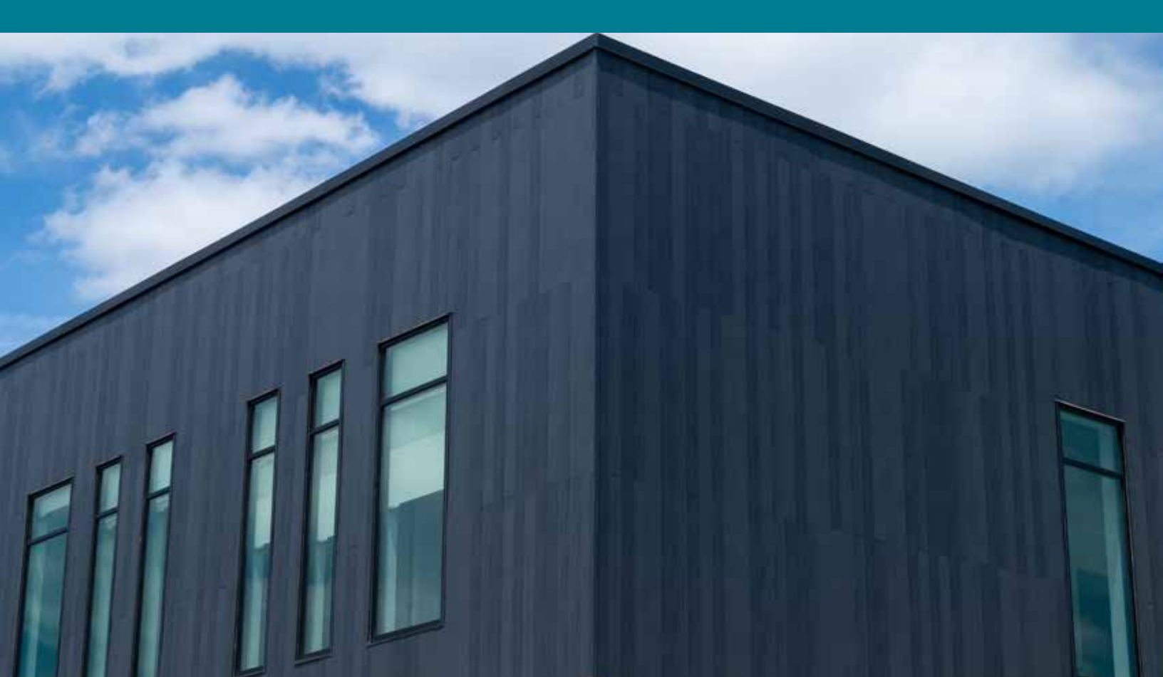
MAC Metal's Harrywood Plus in Black Walnut clads VROC's west- and south-facing façades
